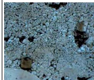
Poor quality concrete – Honeycombing and timber.
