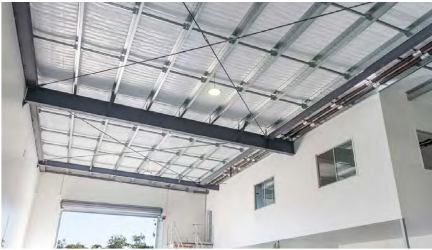
Warehouse featuring Thermoplast white decorative foil sarking
