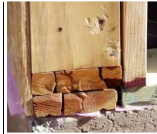
Poor quality timber construction – Split base-plate used.
