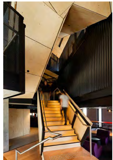
DTAC Ecotac DTO120 and Urban Edging DEO510B installed on a staircase inside RMIT Bundoora West Student Accommodation
