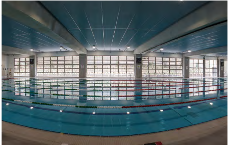
Interior view of the louvre windows that create an impressive floor to ceiling external wall
