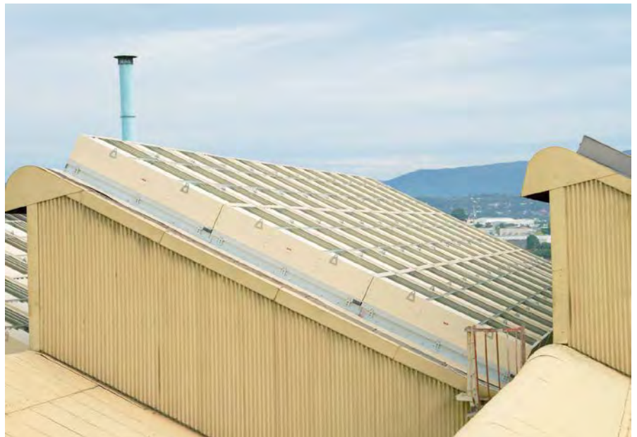
Images of Airocle's installation of the new ventilation system at the BlueScope Port Kembla steel works
