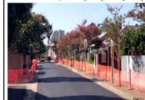
Recycled local road in Sydney
