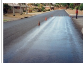
Resealing a local road
