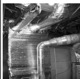
Ductwork insulation.
