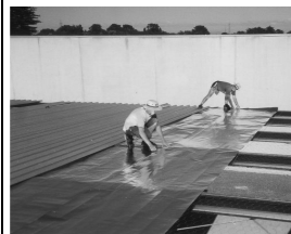
Roof foil insulation.
