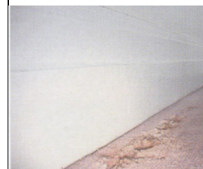
Damage to carpets due to substrate moisture.
