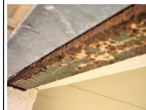
This lintel was revealed during building work on a structure 200 m from salt water and within 2 km of breaking surf.
