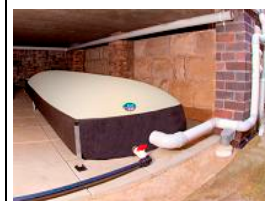
Bladder type tank in sub floor space
