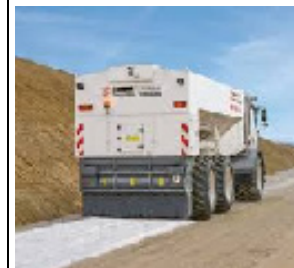
In situ application of binders
