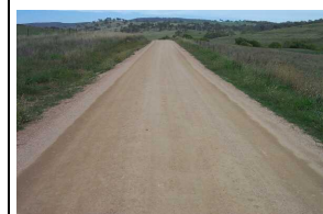
Stabilised unsealed pavement
