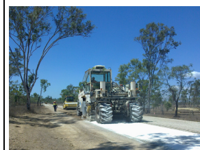
Dry spreading of binders
