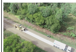
Stabilisation of unsealed pavement in progress
