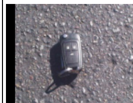
Same age asphalt surface following 3 applications of Enrichment treatment
