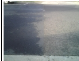
Treated and untreated surface to reduce water infiltration
