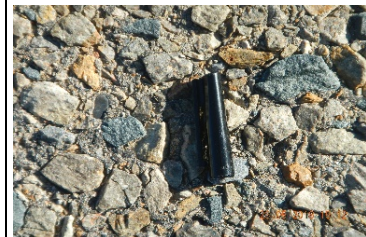
Otta seal stone grading variation
